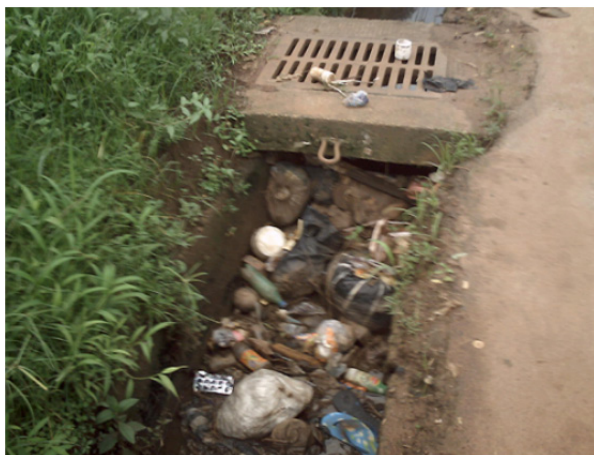
Fig. 7. Solid waste accumulated in the entrance of a manhole of a drainage system
